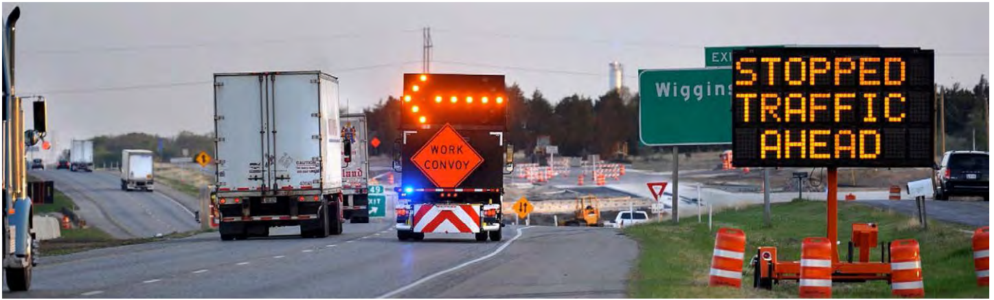
Figure 2. Safety contingency funds have been used for many countermeasures, such as for work zone intelligent transportation systems. (Source: Texas A&M Transportation Institute)
